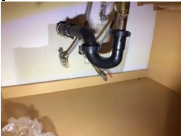
Cabinet Under Sink
