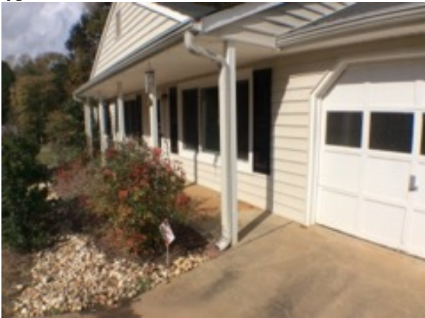
Downspout/Splash Blocks
