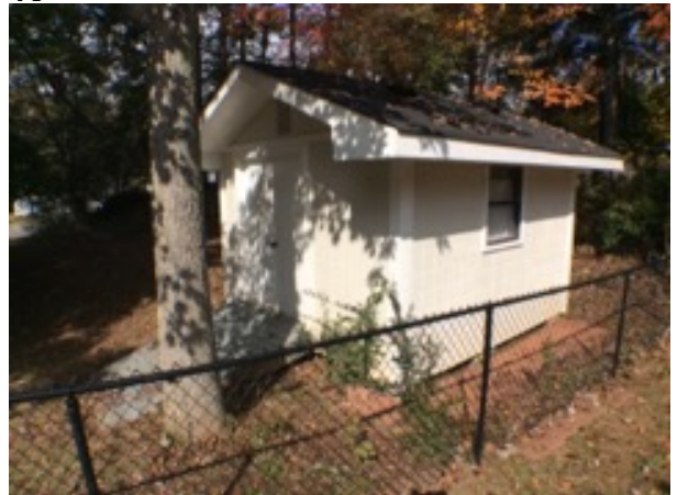
Shed/ Storage Building
