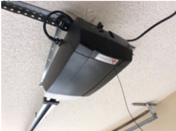
Garage Door Electric Opener
