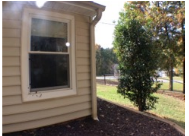
Downspout/ Splash Blocks
