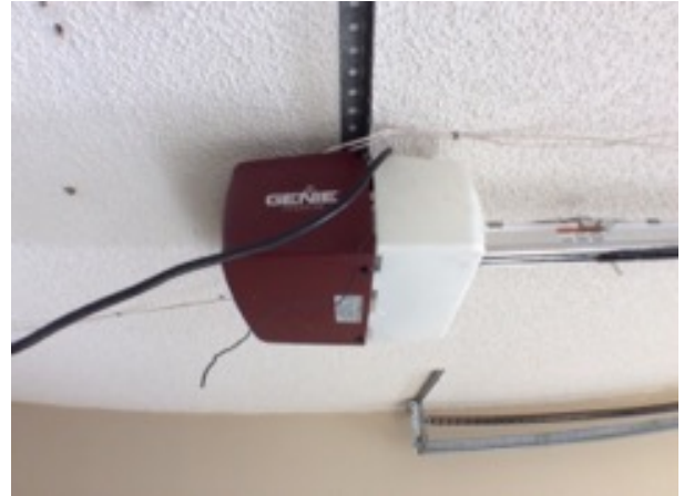
Garage Door Electric Opener
