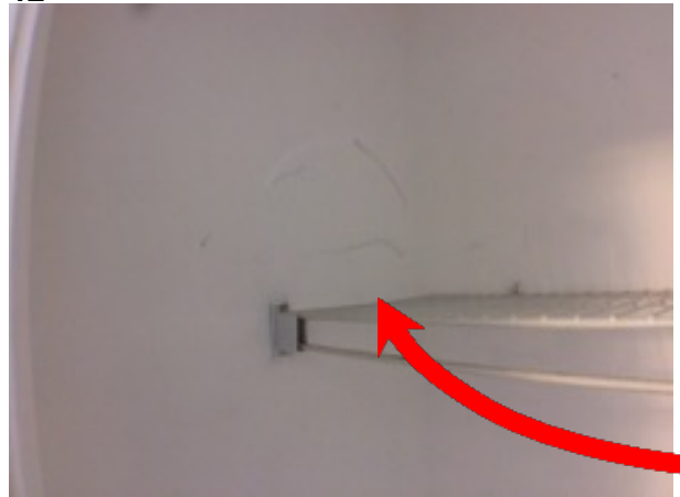
Closets - The walls are marked up.
