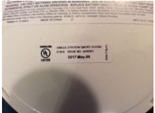
Smoke Alarm (DATE)
