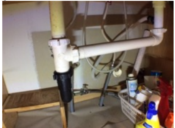
Cabinet Under Sink
